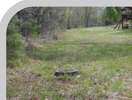
Maintenance of the property within the easement is the responsibility of the property owner.
