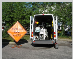
Videoting sanitary sewer lines help prevent spills. We inspected over 72,000 feet of our collection system this fiscal year.
